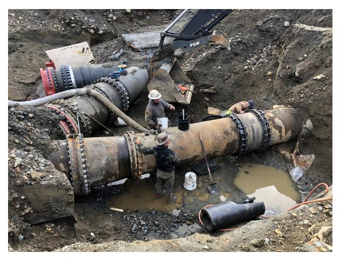
To complete the project BAM LLC is backfilling approximately 1740-feet of abandoned 36 and 24inch water mains with concrete grout to ensure the ductile iron pipes don't continue to corrode to the point of collapsing and causing unexpected substantial subsidence to either the repaved Schoenbar Road or to Walker Field which is due to receive extensive future ballfield improvements including a new layer of synthetic plastic turf.
